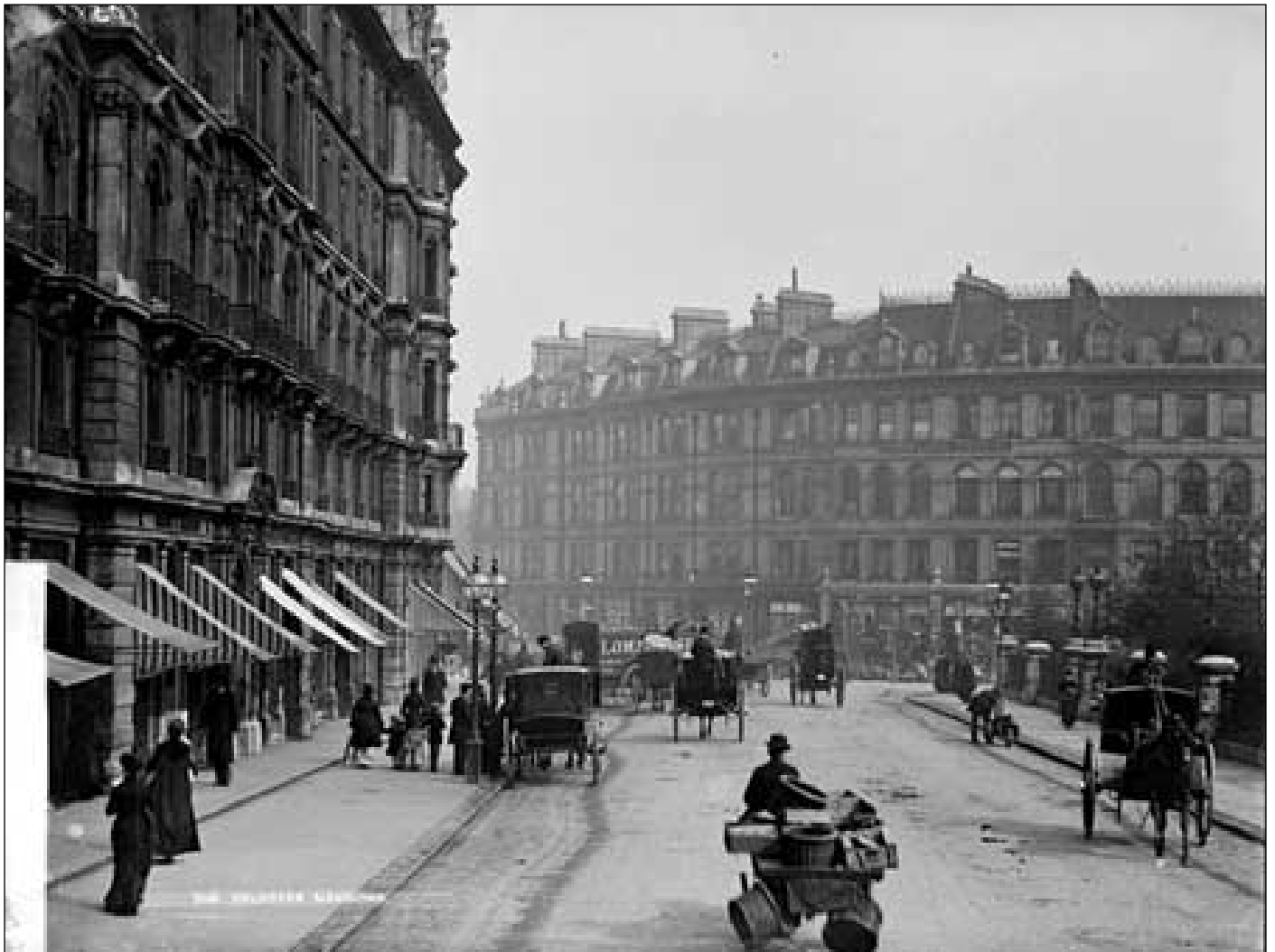
4. Photograph of 23-47 Grosvenor Gardens c.1880. (NMR).
