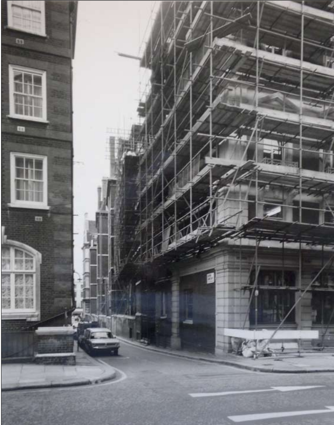
13. Corner of Beeston Place & Eaton Lane 1978 (LMA).
