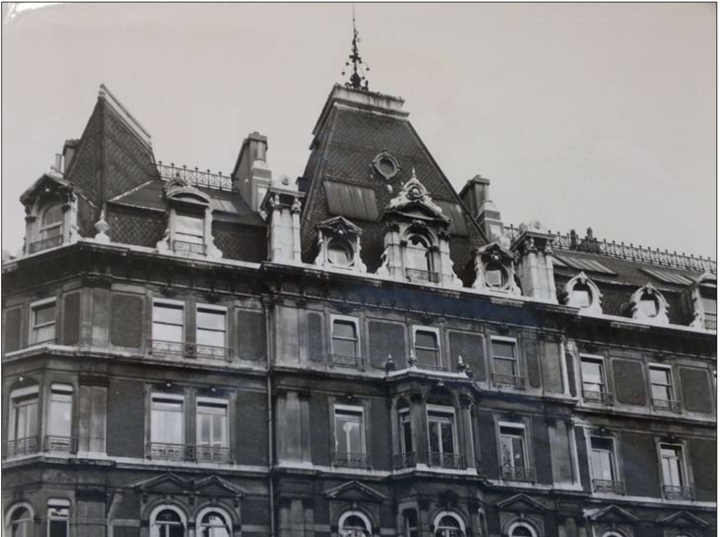
10. Roof detail of 23-47 Grosvenor Gardens 1965 (LMA).
